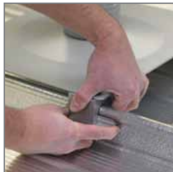
standing seam roof system installation
