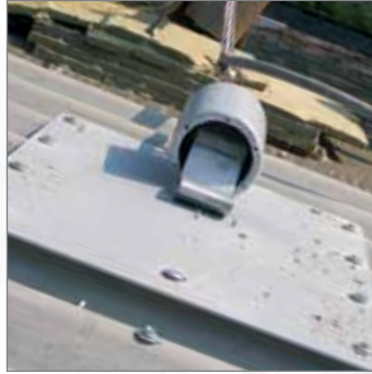
testing the system
