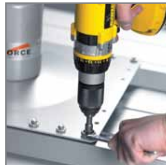
standing seam roof system installation
