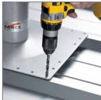
standing seam roof system installation
